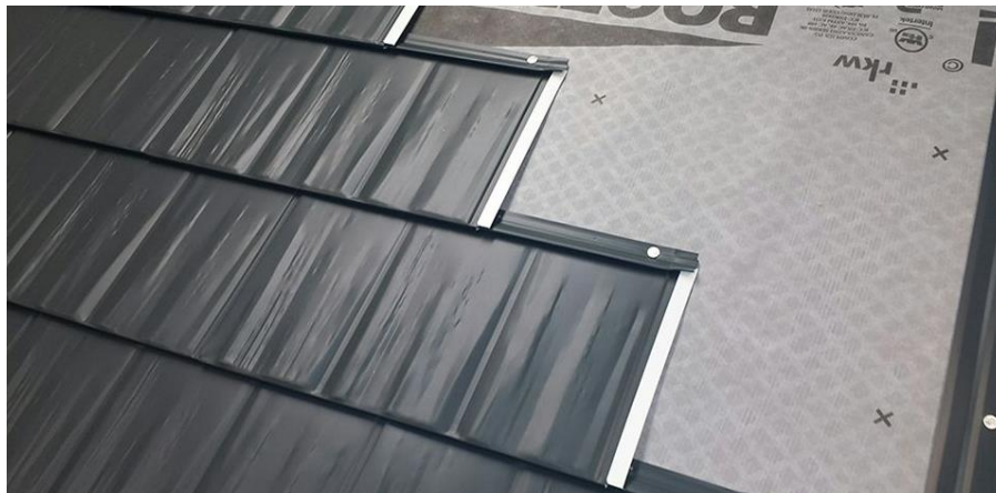
Figure 2 – Cutaway of Metal Shingle roof shows the interlock both horizontally and vertically between the shingles.
