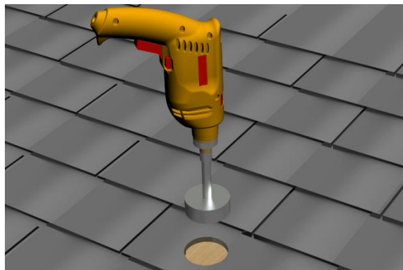
Step 2: Use a 3 inch hole saw to make a clean hole in the metal roof shingle.
