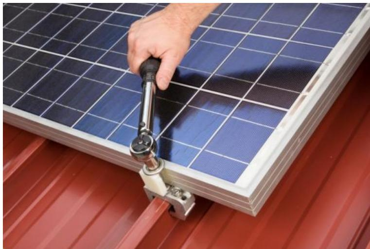
4. Continue to install the AceClamps® ML, Solar-Kits and PV panels in the same sequence for the remainder of the PV array.
