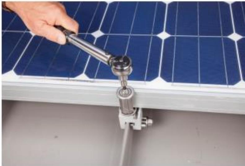
End Spacers are available to match the correct PV frame thickness and are installed at the edge rows to allow the Solar-Kit to be tightened correctly and maintain a neat, finished appearance to your system.
