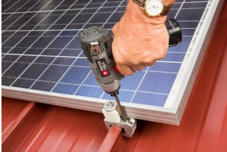
3. Go back to the first row of Solar-Kits and insert the End Spacer and tighten using a 9/16 socket to 100 in. lbs. Torque.
