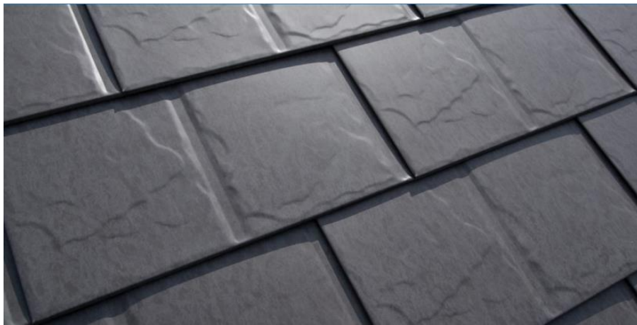
Figure 1 – Typical Interlocking Metal Shingle Roof
