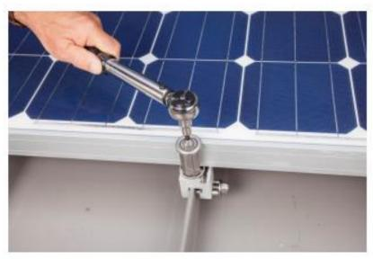
End Spacers are available to match the correct PV frame thickness and are installed at the edge rows to allow the Solar-Kit to be tightened correctly and maintain a neat, finished appearance to your system.
